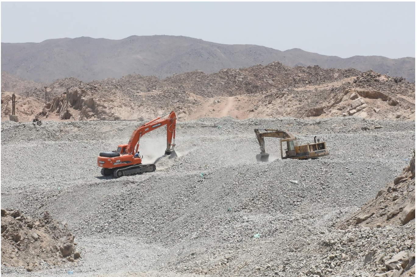
El Sid site – looking east. Recent work on site developing access. Grey rock is the crushed gold-bearing ore.
